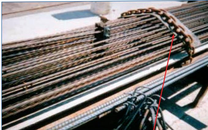
Restraint device installed to prevent cables from releasing in the event of clevis failure during the tension process.
