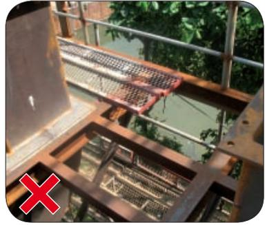
It is important to ensure that boards used for scaffolding are secured. Unsecured boards or planks may shift or even tip over when stepped on.
