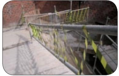
Provide and maintain a guardrail with a lower rail or other effective means to guard open sides of staircases.
