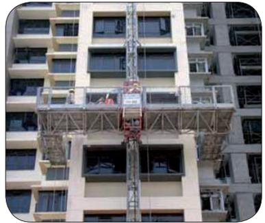
A mast climbing work platform must be installed and used in accordance to its approved design.
