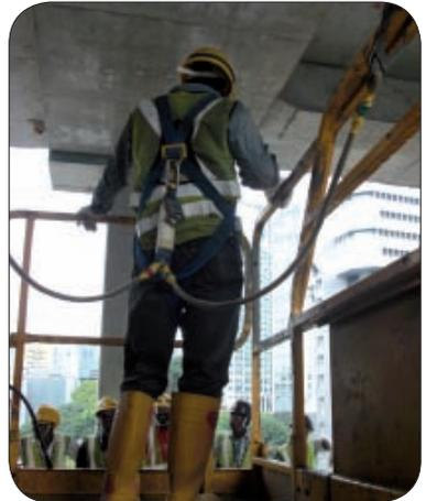
When using mobile elevated work platforms, workers should use safety harnesses with suitable anchorage points.
