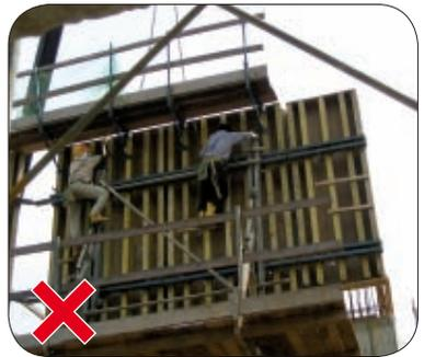
Provide stairs and ladders to enable access from one level of a scaffold to another.
