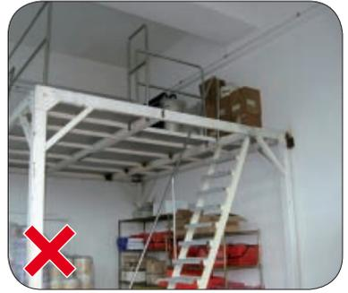
The unguarded open side and staircase are both potential falling hazards. Risk assessment will help identify such hazards in the workplace and control measures that can be used to reduce the risk of falling.
