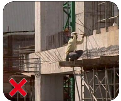
Follow the hierarchy of control: Provide and use correctly other suitable equipment such as safety harnesses or safety belts, only if barricades cannot be provided.
