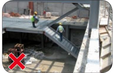
Workers are needlessly exposed to falling risks/hazards if guardrails are not provided on staircases.
